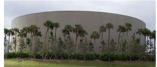
Thermal Energy Storage (TES) Tank
