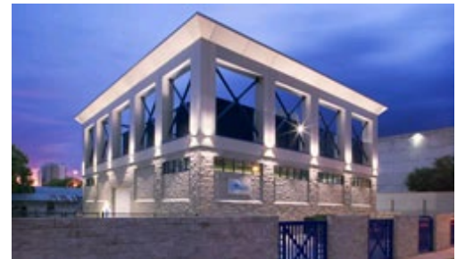
Downtown North CHW Plant
